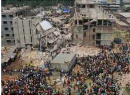
Rana Plaza collapse, 2013
